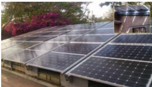
A recently upgraded 9kW<sub>z</sub> Building Integrated Photovoltaic system (BIPV) facility with an inset of indoor natural lighting (Aaditya G and **Mani M**. BIPV: A Real-Time Building Performance Study for a Roof-Integrated Facility. *International Journal of Sustainable Energy*. 2016. 35:1-19).
