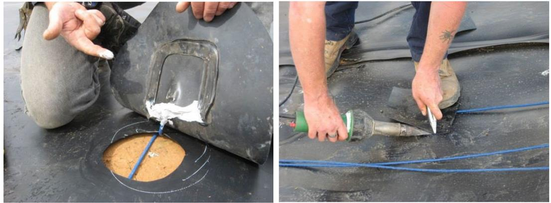
**Figure 4:** A temperature probe being installed in an HDPE pocket beneath the GMB liner above the compacted clay liner at the floor level (left) welding of an HDPE pocket for a temperature probe above the GMB liner at the floor level (right).
