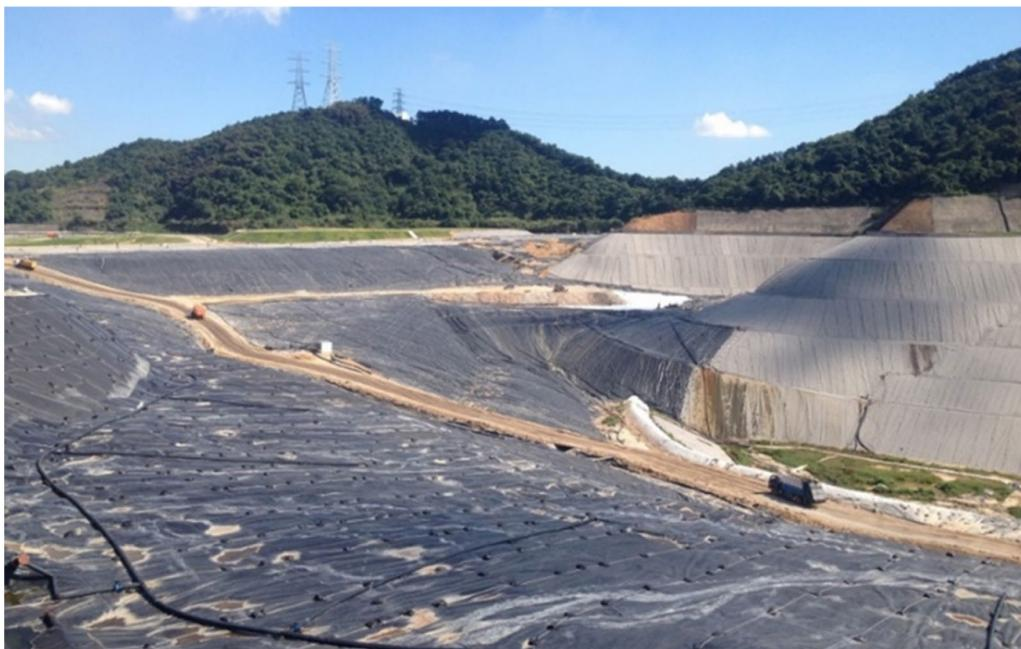
**Figure 15:** A temporary cover and horizontal gas collection wells.
